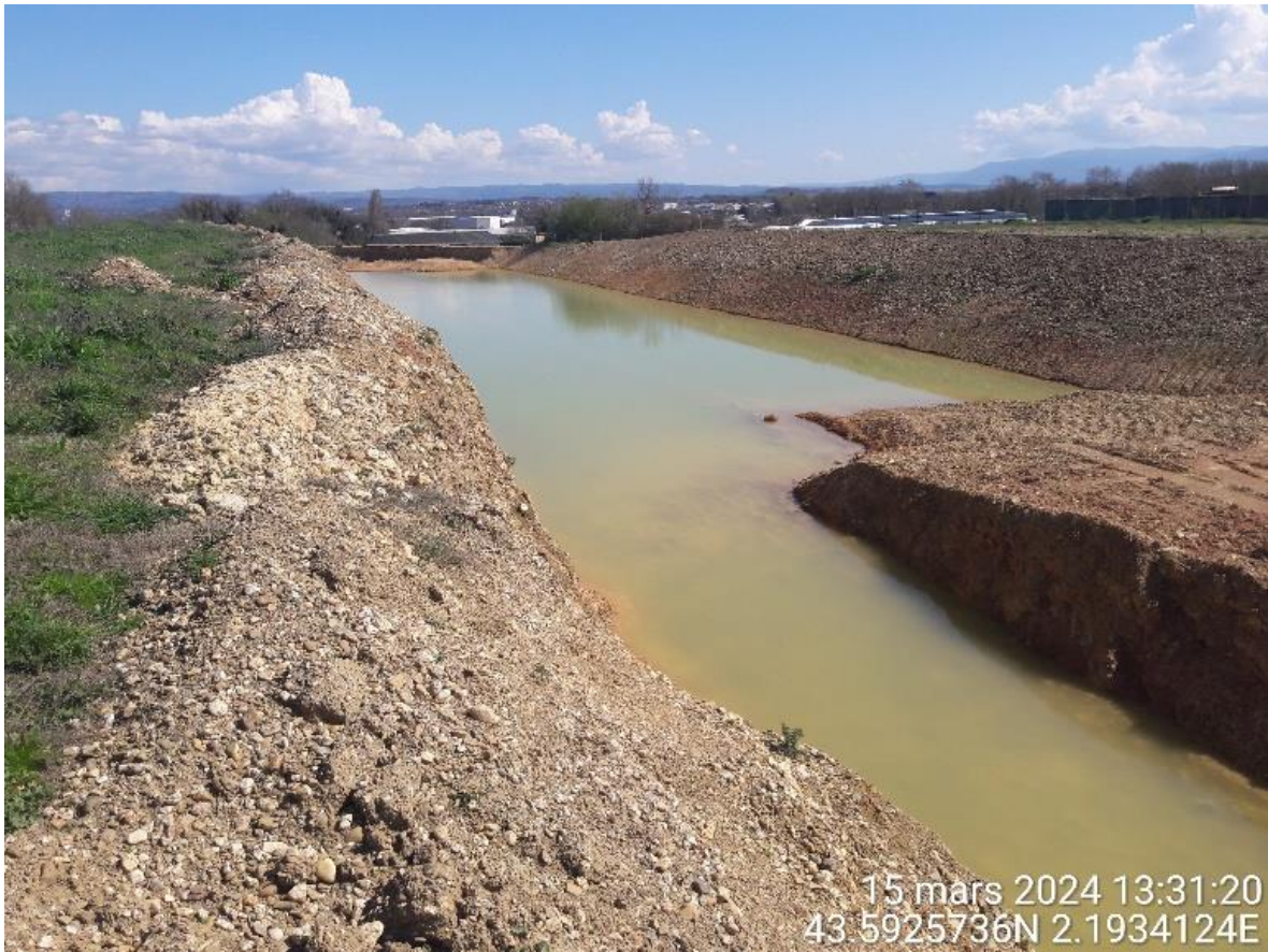
Figure 99: Excavation interception eaux souterraines- CASTRES (81)
