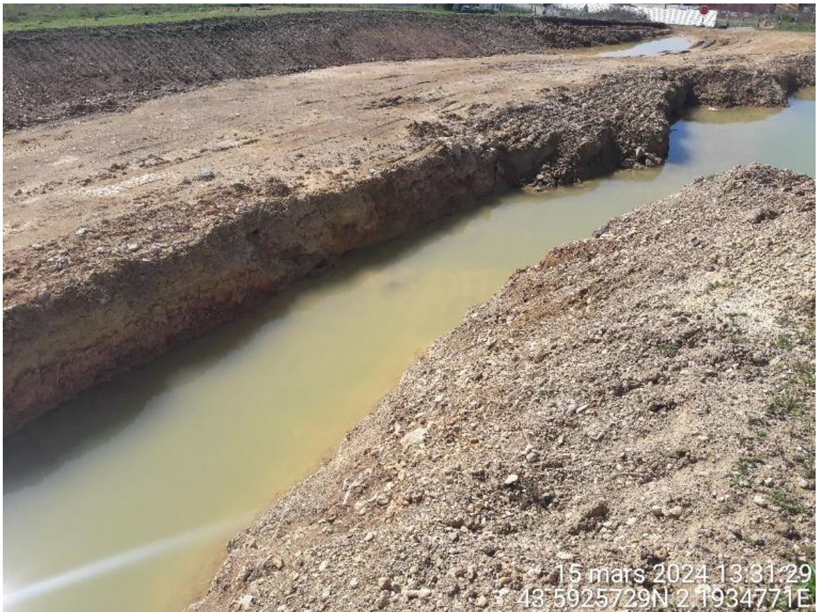
Figure 100: Excavation interception eaux souterraines- CASTRES (81)
